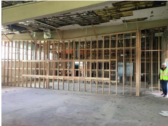
building "A" computer room new wood framing
