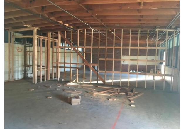
New wood framing in classroom and mechanical room
