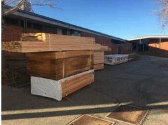
Wood framing preparation and delivery
