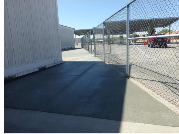
Pathway #2 After Construction
