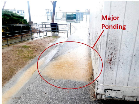
Pathway #3 Before Construction
