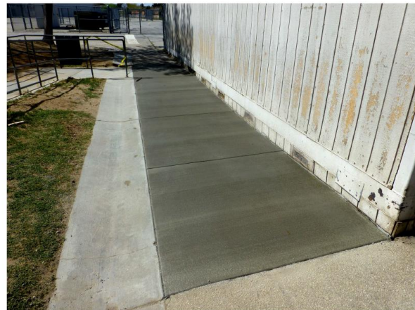
Pathway #3 After Construction (Concrete Sloped to Eliminate Ponding)
