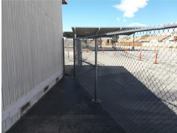
Unsafe Pathway #2 Before Construction
